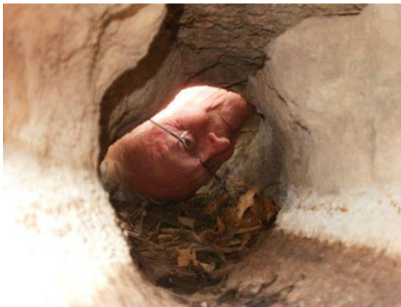
Figure 4. Karst conduit in pure limestone of the Boone Formation showing stain from sediment and water that moved through this void previously. Because groundwater can move so rapidly in karst openings, there is little chance for contaminants to be filtered or attenuated. Flow and transport does not occur continuously in a conduit like this, owing to their great hydraulic conductivity.
